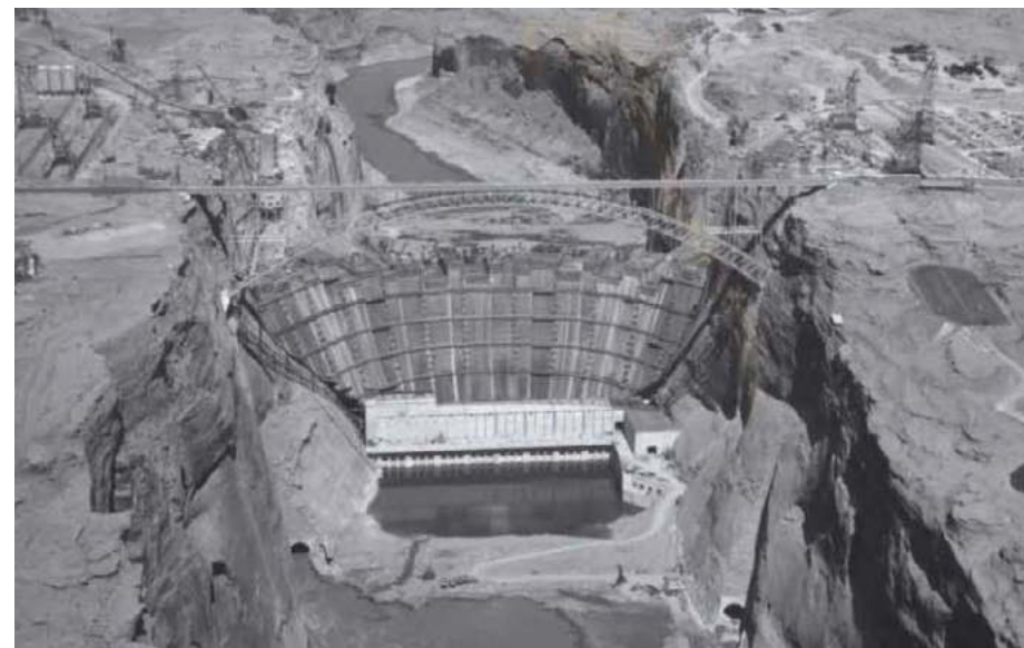
Glen Canyon Dam during construction. Note Colorado River water flowing around the dam at riverbed level through bypass tubes. Photograph from Bureau of Reclamation.
