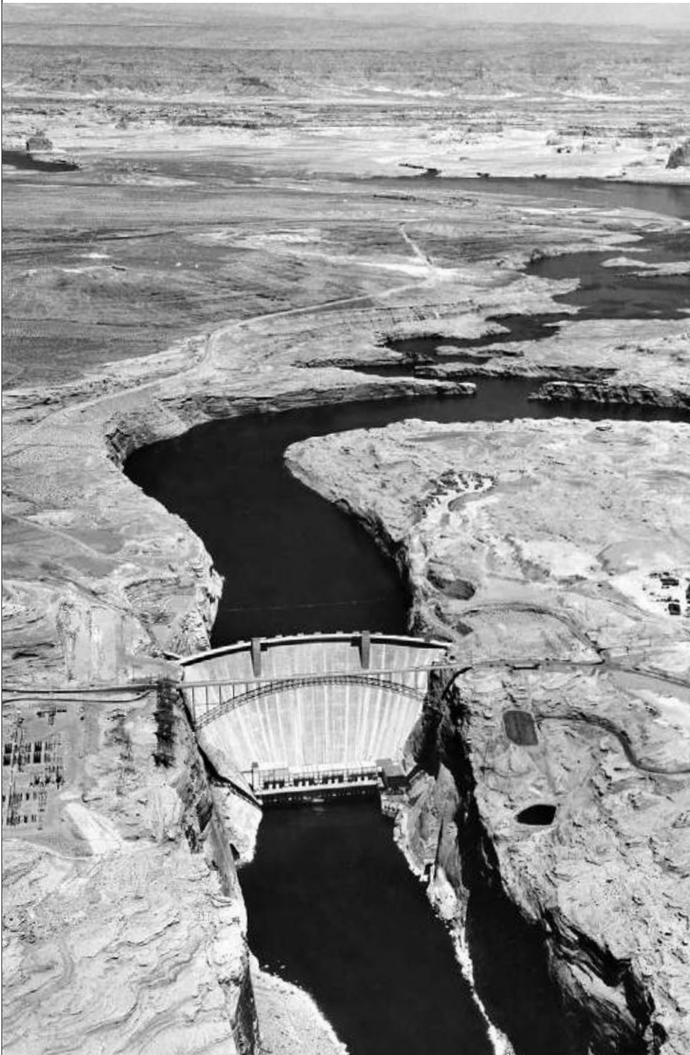
Glen Canyon Dam during construction. Note Colorado River water flowing around the dam at riverbed level through bypass tubes. Photograph from Bureau of Reclamation.
